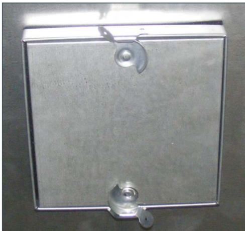
Nominal size: 200mm × 200mm (access panel 195mm × 195mm)
